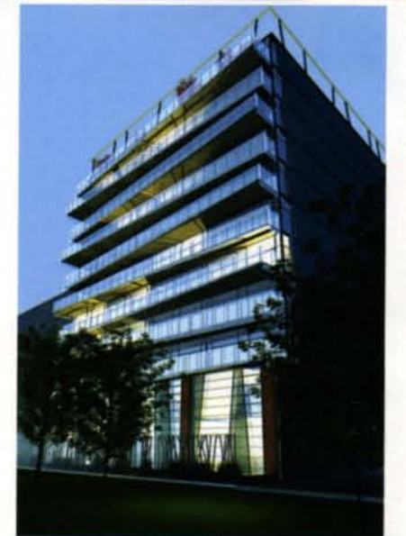
Parc Lofts – the latest addition to LDC’s portfolio, is an intimate loft building backing onto a park in the heart of King West.
